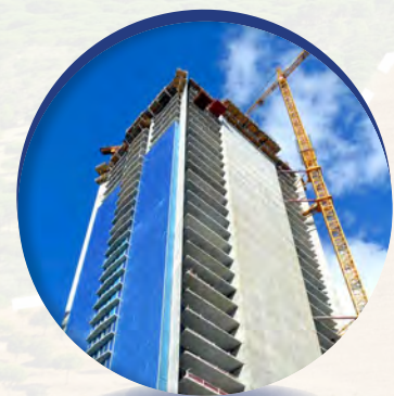
HOUSING SOCIETIES CONSTRUCTION
